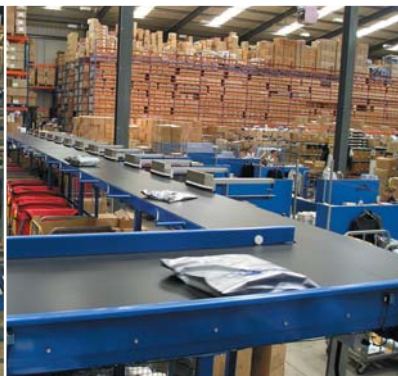
Belt Conveying Systems
